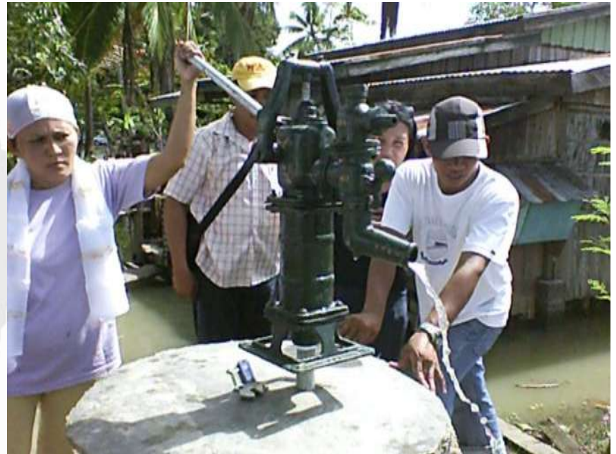
Improved Dug Well and Pump installation and repair Training Kabuntalan, Maguindanao Feb 2009
