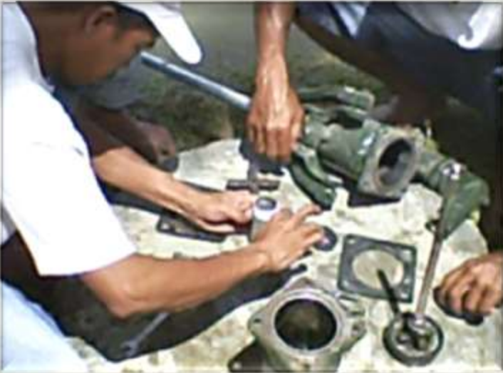
Hand Pump Repair ← Dug Well Improvement →
