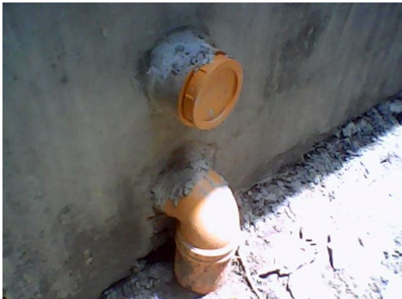
Clean out port and discharge to Leach Field
